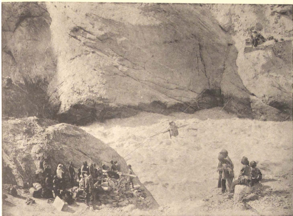
a. Crossing the Spiti River by a rope bridge.
