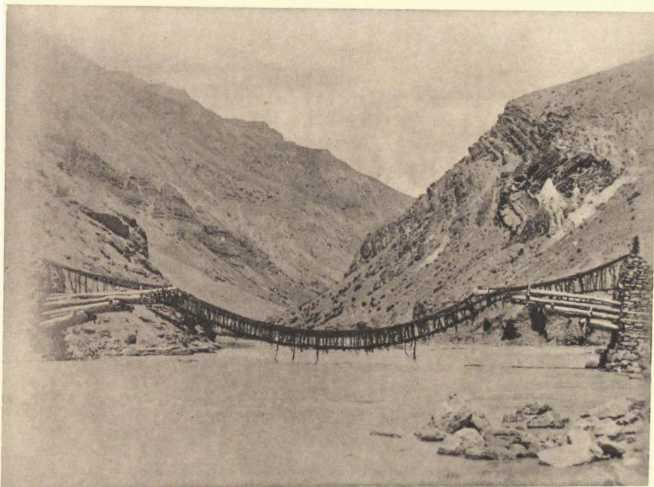
b. Rope bridge near Lithang.
